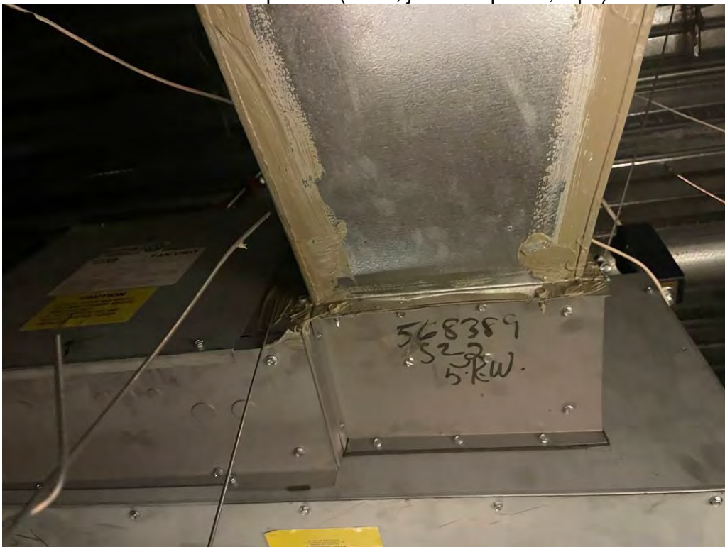
Photo 4: Non asbestos containing duct sealant.
