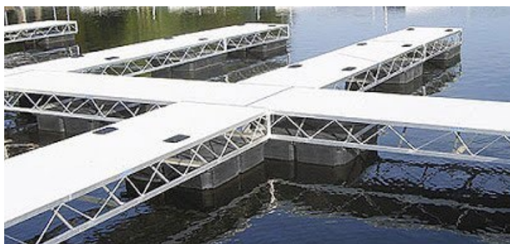
Figure 39: Docks built on floating blocks.
