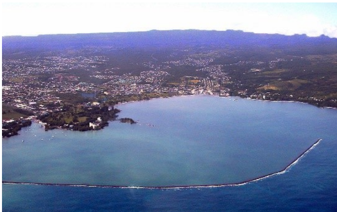
Figure 45: Breakwater protecting the harbor in Hilo, Hawaii built far out from harbor area.
