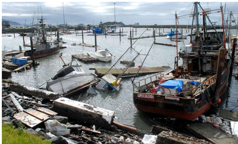
Figure 2: Damage in Crescent City, California, from the 2011 Japan tsunami, about 10 hours after the initial earthquake.
