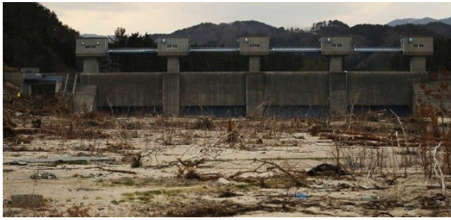
Figure 44: Floodgates in Fudai, Japan.
