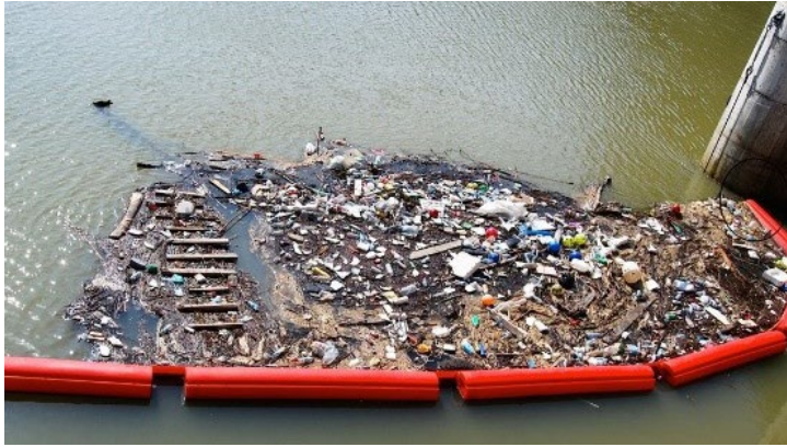
Figure 47: Debris deflection boom.
