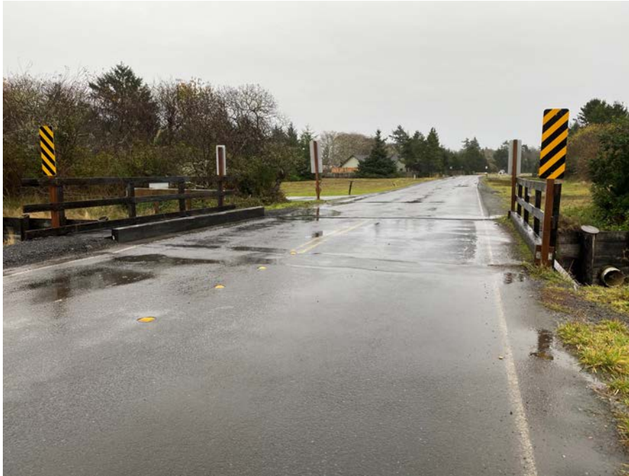
East Chance a La Mer Northeast (looking east)
