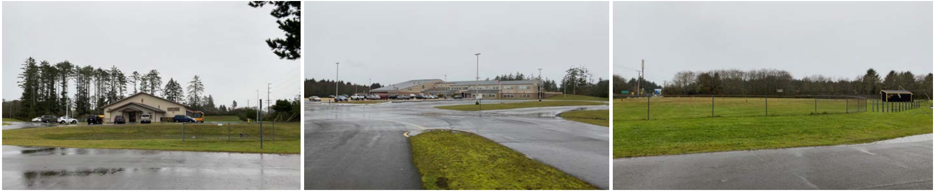
OSW 4 - North Beach Junior/Senior High School (from left to right: admin building, school, sports field)
