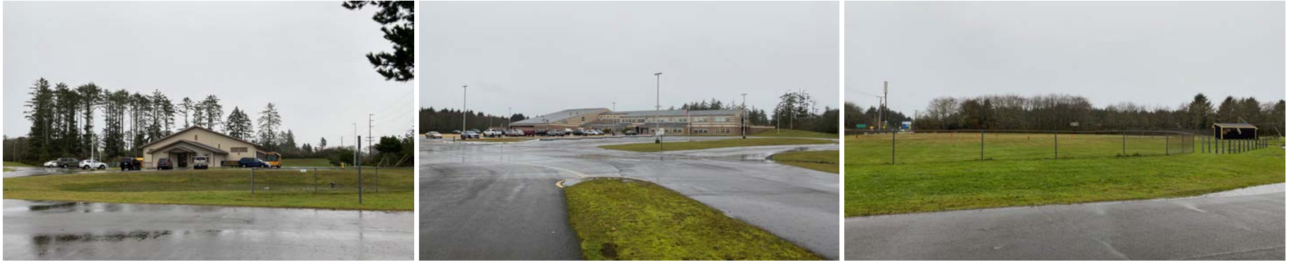
OSW 4 - North Beach Junior/Senior High School (from left to right: admin building, school, sports field)
