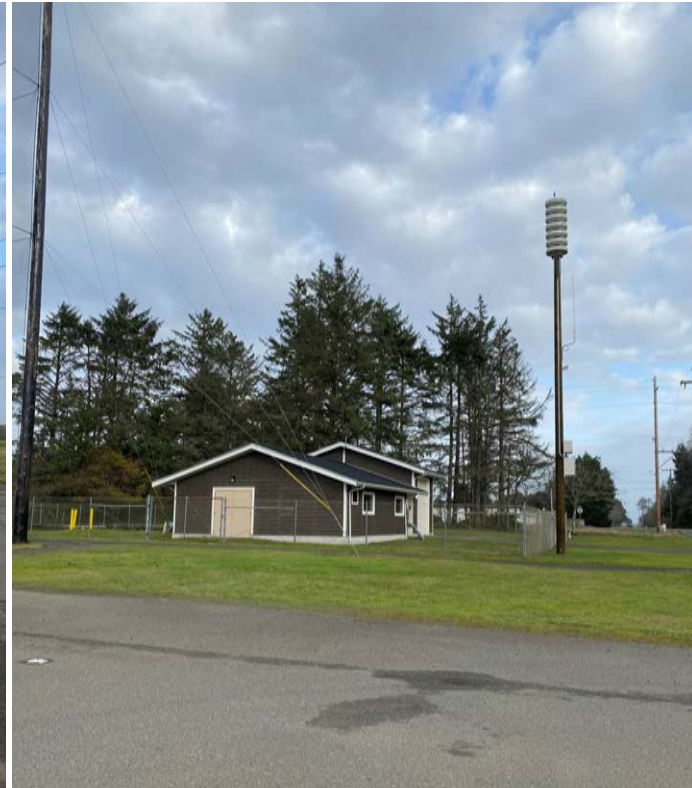
OSE 1 - AHAB siren site Photo Credit: Jeana Gómez
