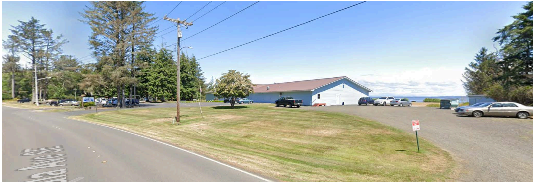
OSE 8 - Alternative #2 : Ocean Shores Community Club-owned property just north of OSE 8. Lots of open space that could potentially accommodate a VES tower.
