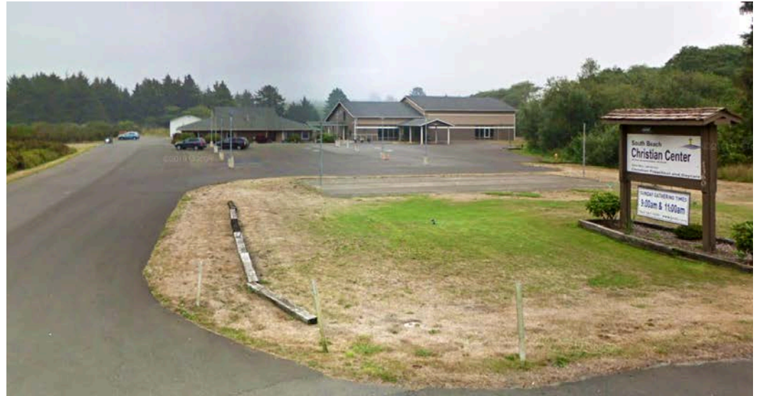
G 4 - South Beach Christian Center parking lot, view from street
