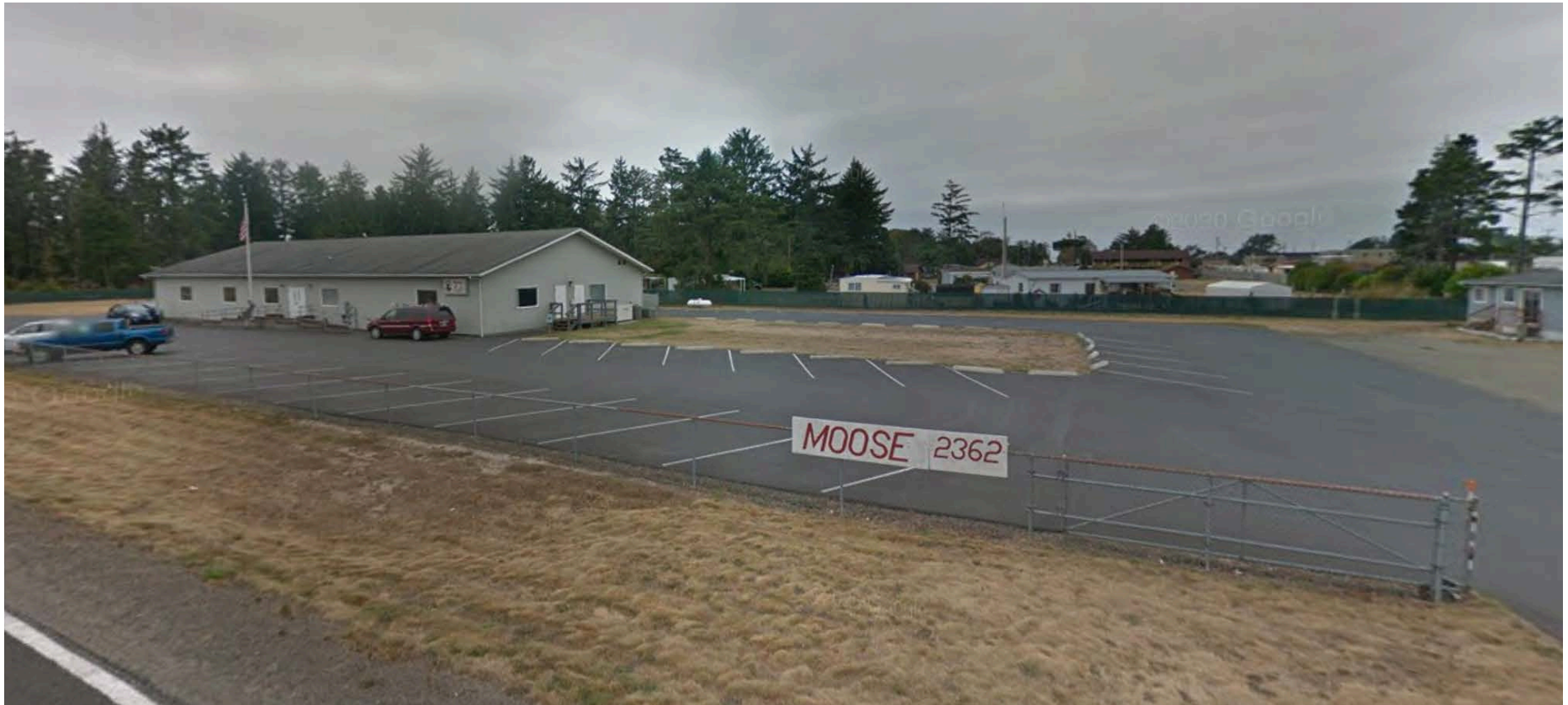
OP 5 - Alternative #1 : Moose Lodge, large parking area
