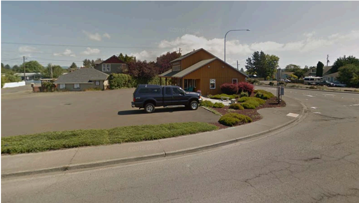
S 1 - Alternative #1 : Nearby, State of Washington-owned parcel with Tourism Bureau building on SR 103.
