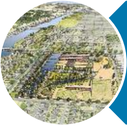
Mirabeau Water Garden, New Orleans, LA
