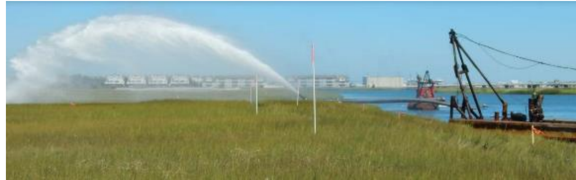
Coastal wetlands restoration, Middle Township, NJ
