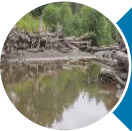
Calistoga Reach Levee Setback and Side Channel Construction, Pierce County, WA
