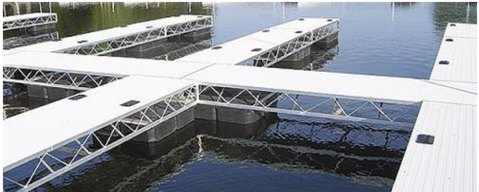
Figure 46: Dock built on floating blocks.
