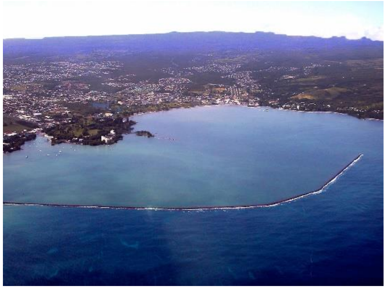
Figure 51: Breakwater protecting the harbor in Hilo, Hawaii built far out from harbor area.
