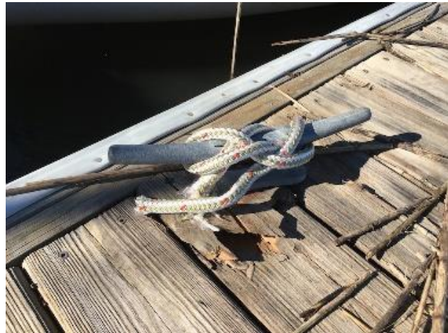
Figure 30: Cleat ripped from dock.
