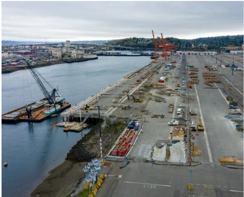
Figure 40: Wharf construction at the Port of Tacoma.
