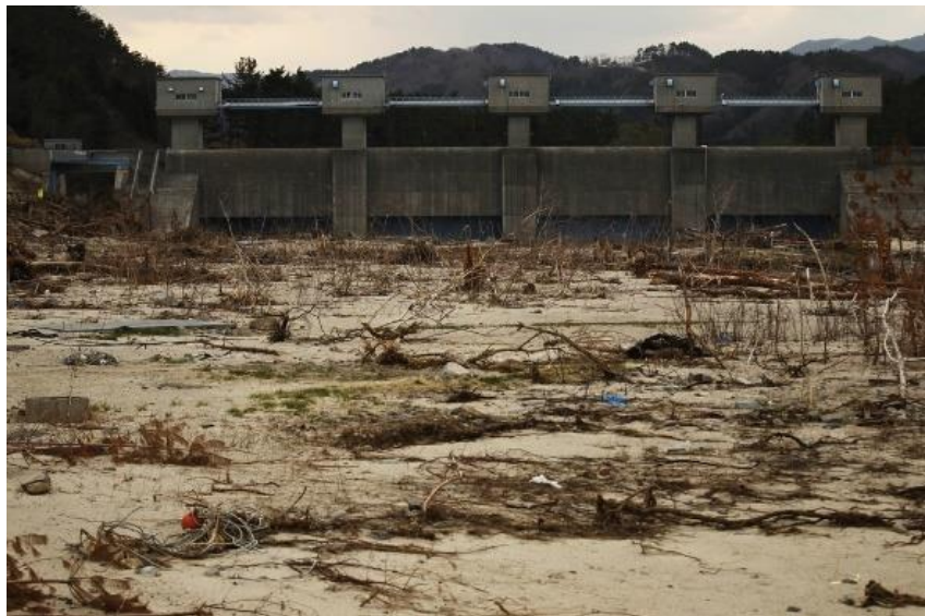
Figure 50: Floodgates in Fudai, Japan.
