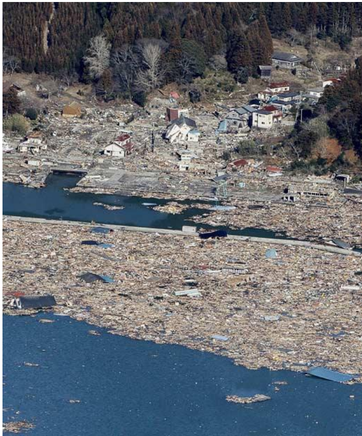
Figure 5: Tsunami debris in the water after 2011 tsunami in Ishinomaki, Japan. Koyodo News / AP
