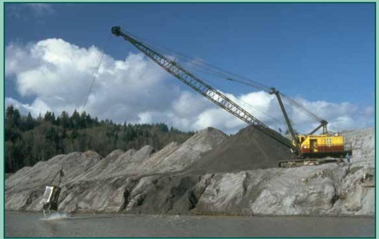
The U.S. Army Corps of Engineers dredged extensively to restore the channels of the Columbia River for navigation and the Toutle and Cowlitz Rivers for flood control. Piles of dredged debris remain visible along Interstate 5. U.S. Geological Survey photograph by Lyn Topinka, February 5, 1981.
