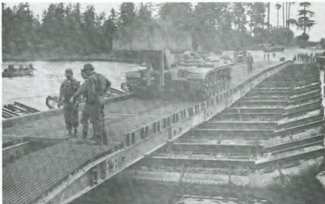
During annual training, the 286th Engineer Company (Bellingham and Anacortes) completed a Pontoon Bridge across Lake Sequelitchew.
