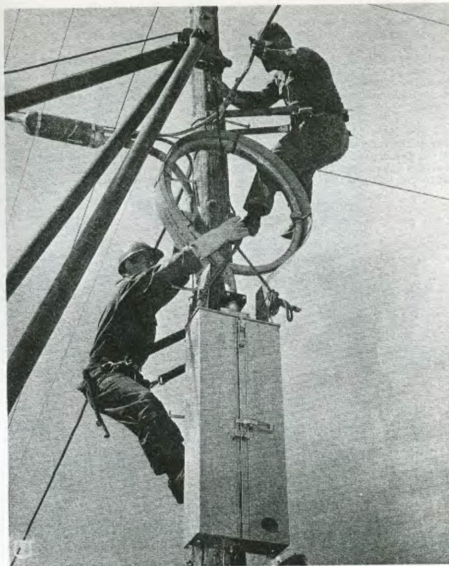
Personnel of the 215th Electronics Installations Squadron installing a telephone system.
