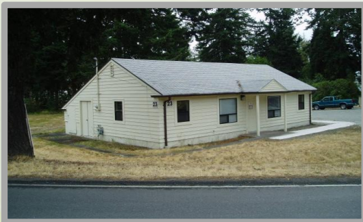
Bldg. 23 at Camp Murray before renovation
