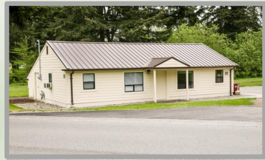
Bldg. 23 at Camp Murray after renovation
