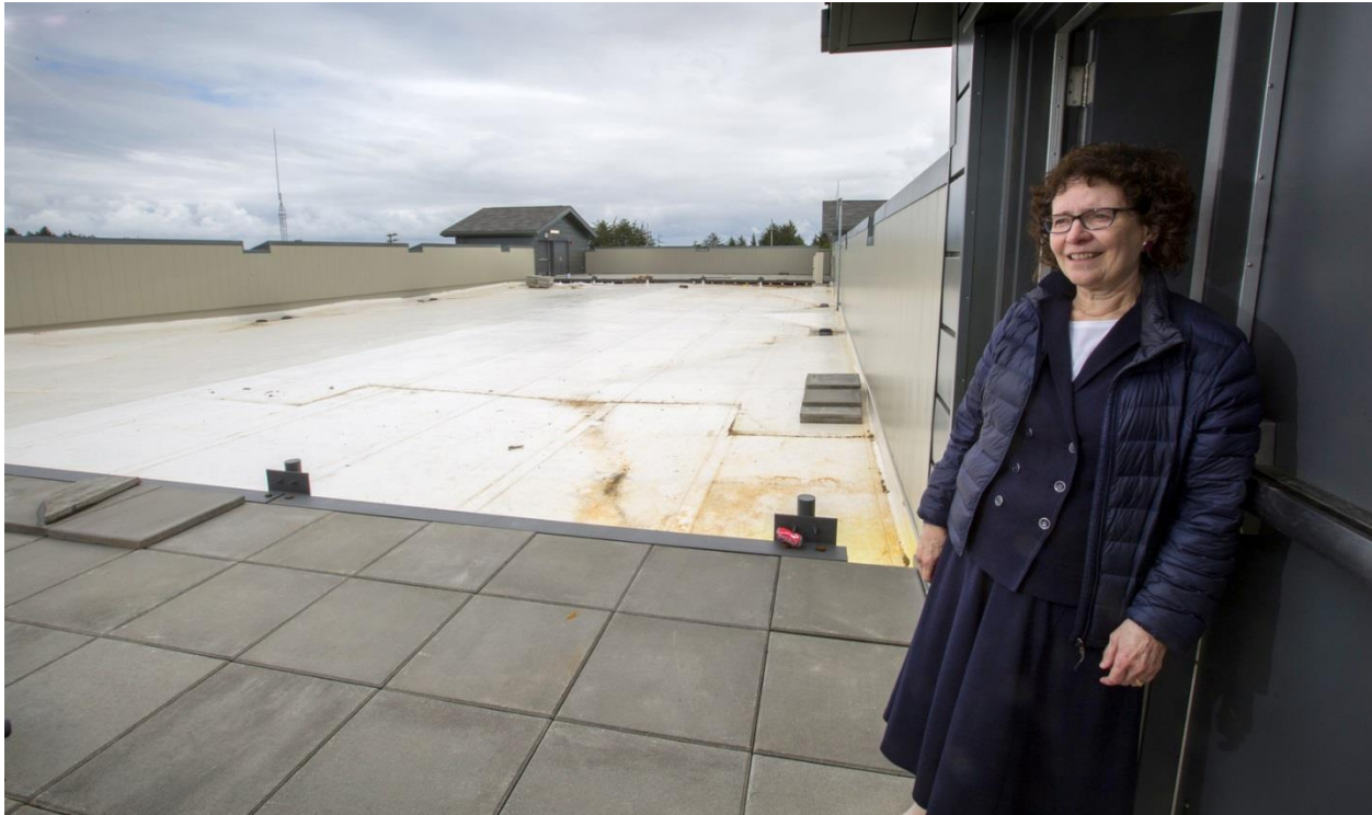
Paula Akerlund, superintendent of the Ocosta School District on the Washington Coast, was instrumental in turning the dream of a safe-from-tsunami Ocosta Elementary School building into reality. She is standing on the gym rooftop, which can be a haven for at least 2,000 people. (Ellen M. Banner/The Seattle Times)
