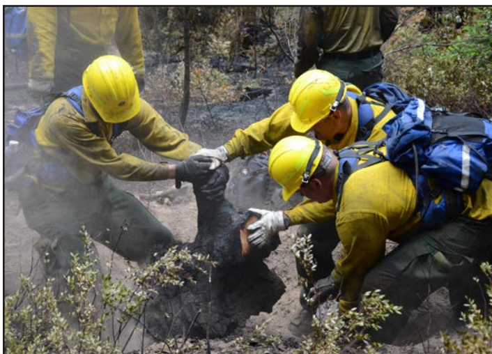
Guardsmen, with the 1-303rd Cavalry Regiment, remove a tree stump while clearing an area recently affected by the Chiwaukum Complex wildfires near Leavenworth, Wash on July 23, 2014. Guardsmen must remove large stumps like this one to ensure there are no remaining embers beneath that could reignite fires. (Photo by Washington Army National Guard Pvt. Brianne Patterson)
