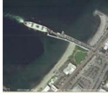
Edmonds Ferry Terminal
