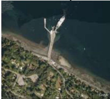
Vashon Island Ferry Terminal
