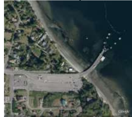
Southworth Ferry Terminal
