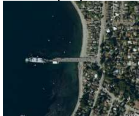
Fauntleroy Ferry Terminal
