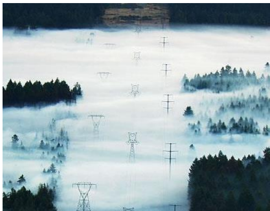
Figure 5.5-5 Smoke from Powerline 2 Fire, DNR 2012
