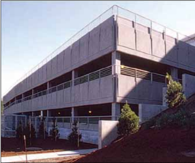
Figure 8: Building for vertical evacuation. Buildings can be used for other functions when not needed for evacuation.
