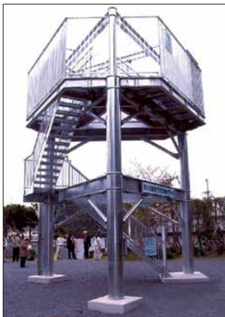
Figure 6: Basic tower This metal tower is used in Japan.
