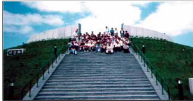
Figure 5: Constructed berm with stair access
