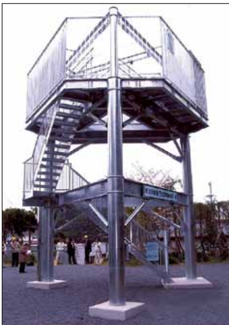
Figure 6: Basic tower for tsunami refuge This metal tower is used in Japan.
