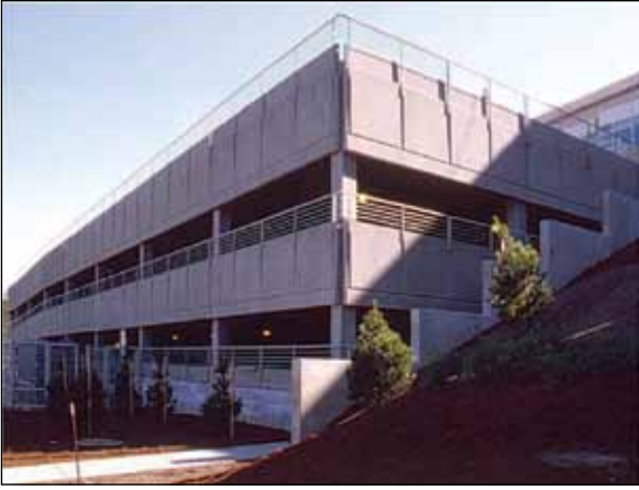
Figure 8: Building for vertical evacuation. Buildings can be used for other functions when not needed for evacuation.
