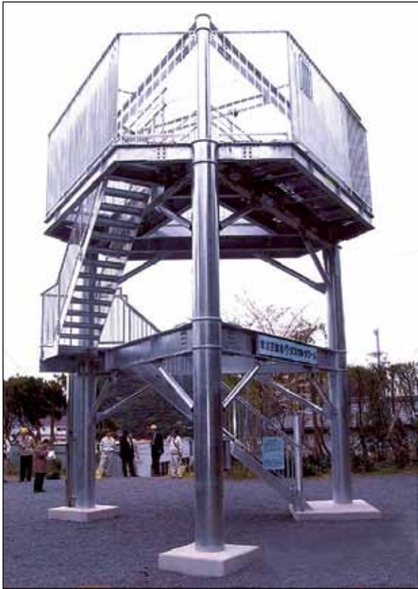
Figure 14: Basic tower for tsunami refuge This metal tower is used in Japan and this type of structure was important in saving lives in the 2011 Tohoku tsunami.
