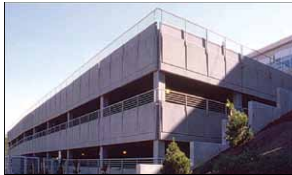
Figure 15: Building for vertical evacuation Buildings can be used for other functions when not needed for evacuation. Parking garages are one option as well as other building with specific areas built to withstand tsunami forces.
