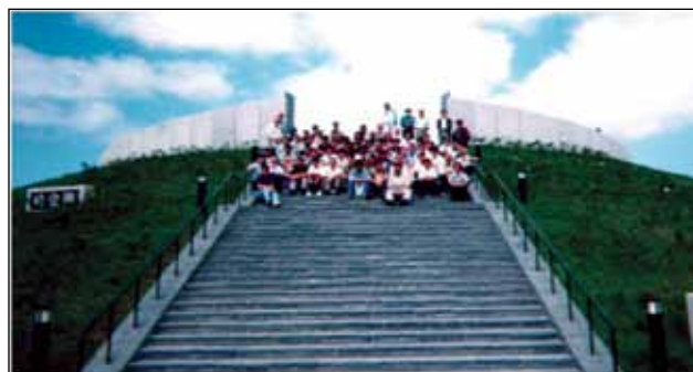
Figure 12: Constructed berm with stair access
