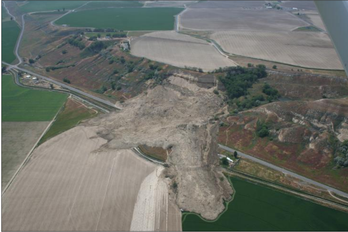
Figure 8. At about 9 p.m. on Saturday, May 13, 2006, a large section of bluff sloughed off and covered about a quarter-mile of Road 170 to a depth of about 40 feet. Photo courtesy of the South Columbia Basin Irrigation District.
