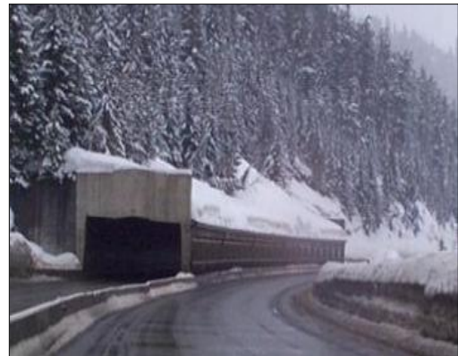
Snow shed over Interstate 90 Westbound
