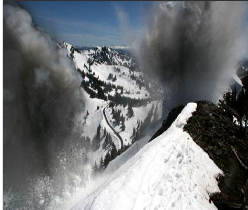
Use of explosives to prematurely trigger avalanche on Chinook Pass
