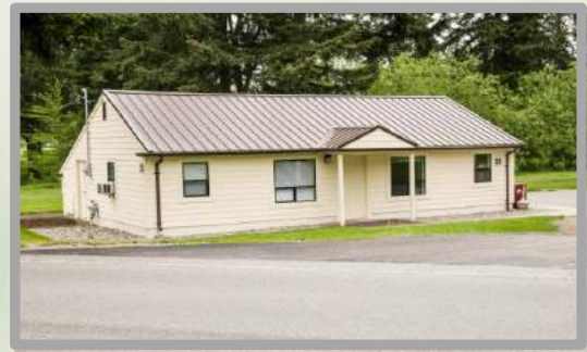
Bldg. 23 at Camp Murray after renovation
