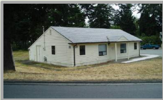
Bldg. 23 at Camp Murray before renovation
