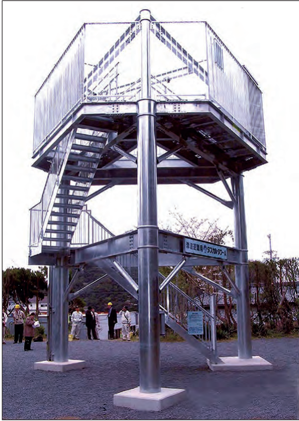
Figure 11: Basic tower for tsunami refuge This metal tower is used in Japan and this type of structure was important in saving lives in the 2011 Tohoku tsunami.
