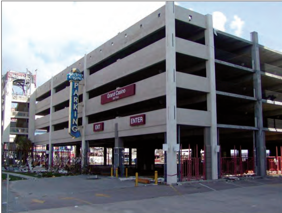
Figure 12: Building for vertical evacuation Cast-in-place reinforced concrete parking garage in Biloxi, Mississippi after hurricane Katrina. Open structural systems allow water to pass through with minimal resistance, and interior ramps allow for easy ingress and vertical circulation.
