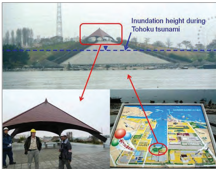
Figure 10: Constructed berm Soil berm combined with a community park at Sendai Port, Japan. Concrete lining on the ocean face can deflect incoming waves while sloped sides provide for quick access.
